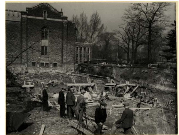
Photographer: Unknown Construction of Emmanuel College, 1930 1991.161/547 Victoria University Archives
